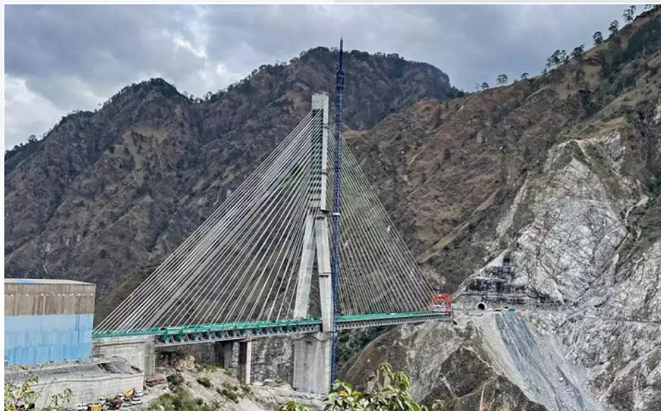
Anji Khad Bridge
